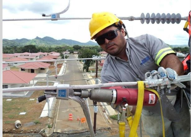
We are pleased to announce the introduction of our new line of battery actuated WEJTAP connector installation tool. These self contained battery powered WEJTAP hydraulic tools use a combined proven platform of WEJTAP tool heads and 18volt Ni-MH battery hydraulic tools to offer a reliable WEJTAP Tool that does not require explosive booster cartridges!
